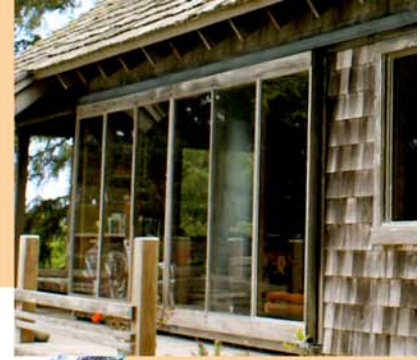
SOUTH WINDOWS, WITH TILE FLOORS, CAN BE AN INEXPENSIVE WAY TO HEAT A HOME.
