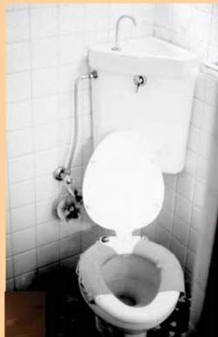
WISE APPLIANCES SAVE IN MANY WAYS. HERE A CORNER TANK DUAL-FLUSH TOILET WITH HANDWASHING SINK IN THE LID.
