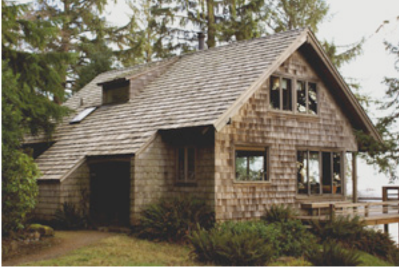
Left: Woodshed and entry porch are on the north, out of the coastal winds.
