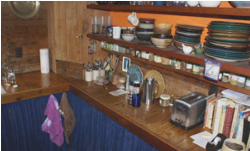
Left: Kitchens and other interior areas can be left "unfinished", with homeowner doing finish work. This kitchen cost $100, including recycled stove and sink, and a "cool box" rather than a refrigerator. Towel "curtains", 2x12 shelves, and counters made from ends of flooring saved money.
